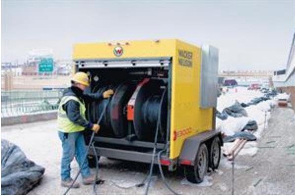
*One way to fight back against the cold is with hydronic heaters that circulate hot water through flexible hoses.*
