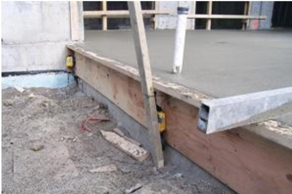
*Maturity meters provide a simple way to determine concrete strength.*
