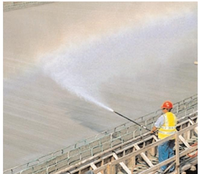
**Fig. 13-11.** Fogging cools the air and raises the relative humidity above flatwork to lessen rapid evaporation from the concrete surface, thus reducing cracking and improving surface durability. (69956)
