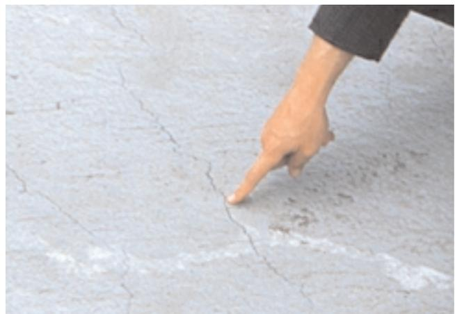
Fig. 13-7. Typical plastic shrinkage cracks. (1311)
