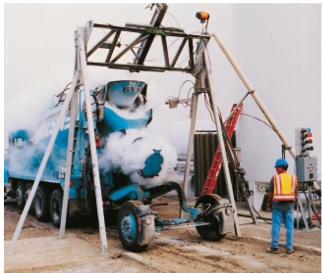
**Fig. 13-1. Liquid nitrogen added directly into a truck mixer at the ready mix plant is an effective method of reducing concrete temperature for mass concrete placements or during hot-weather concreting. (69954)**
